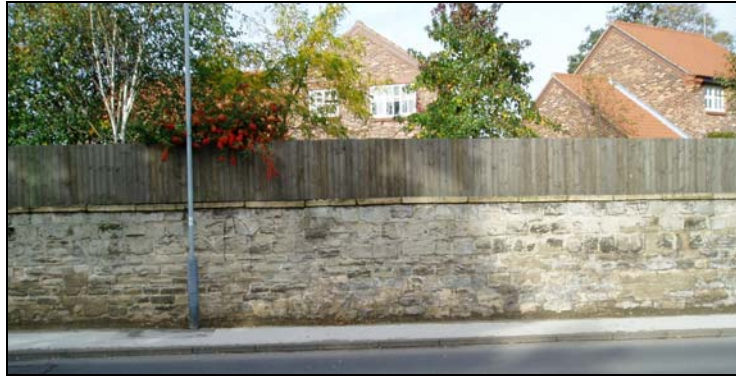
Old Hall Close boundary wall
