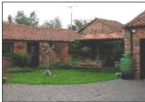
Outbuildings still in use
